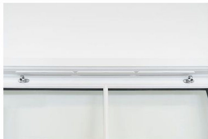
Internal View (vents closed)
