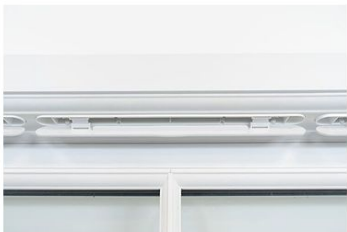
Internal View (vents open)
